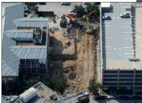
Aerial view of CAC Expansion
